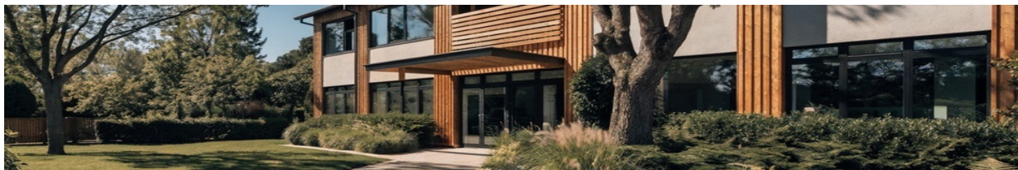
These questions apply to any building with a water system — where you live, work, stay or visit. Illustrative image.
